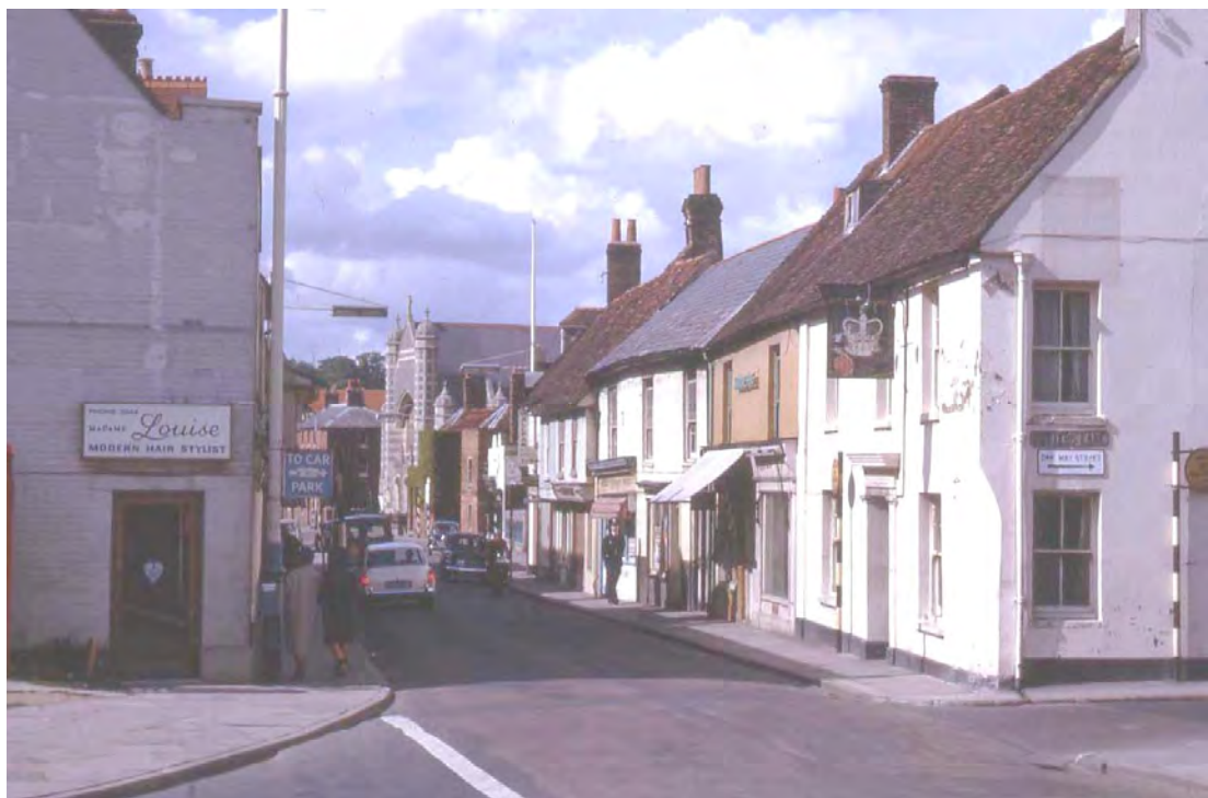
Church Street with the junction with Potters Lane on the right. All the buildings shown have been demolished.
